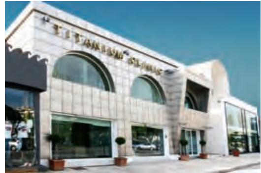
The façade of the Titanium Clinic in Marbella is covered with 100 two-millimetre titanium plates.
